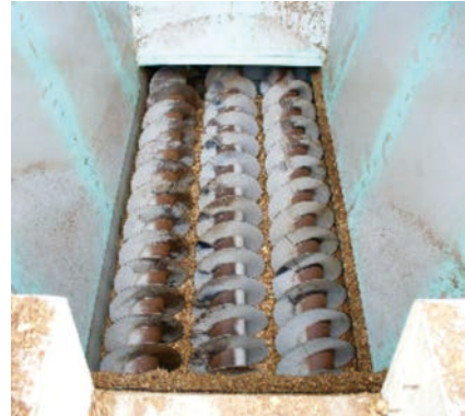
Mounting in discharge screw (wood-fired power plant)
